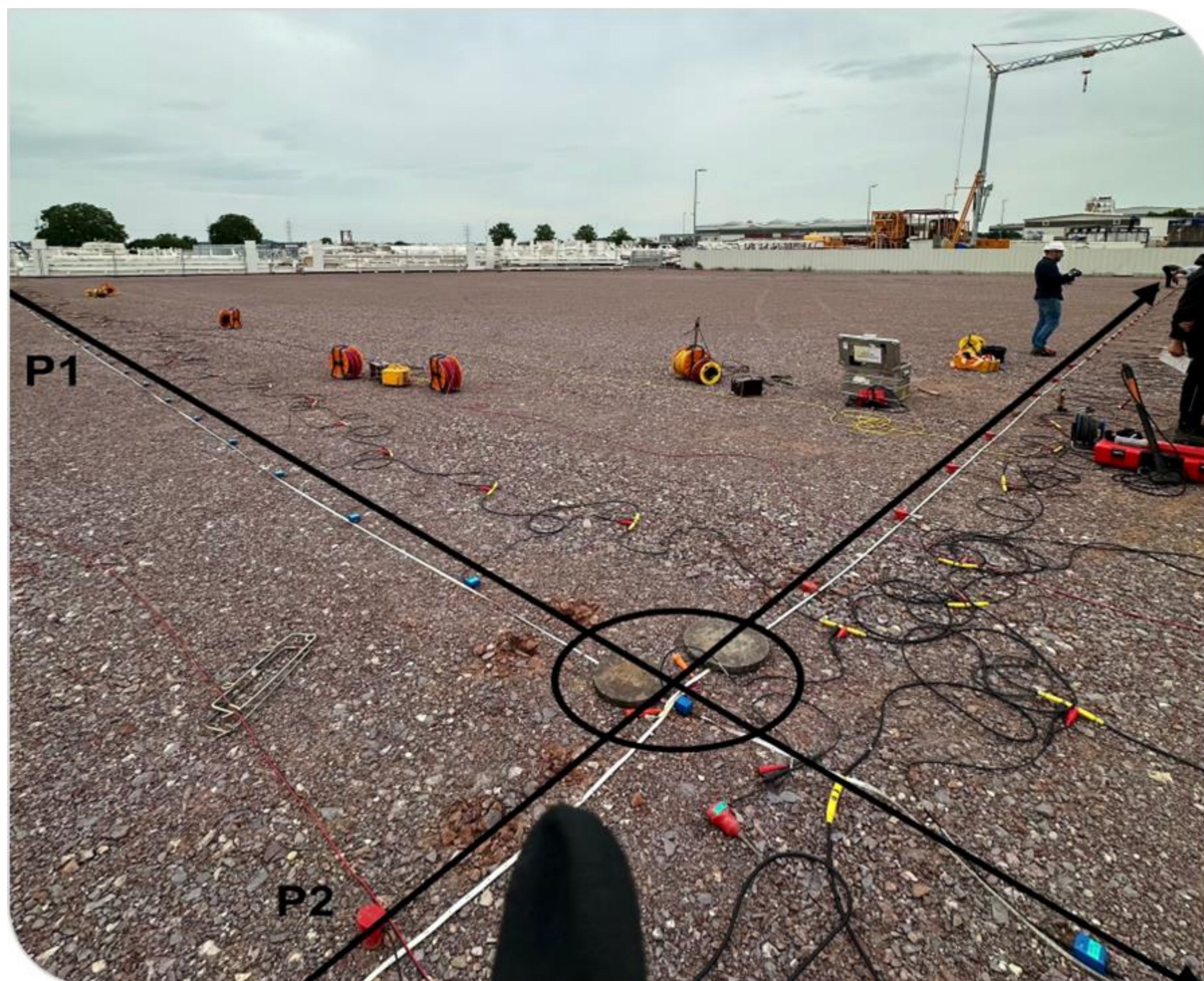
Figure 2: View of the two orthogonal measurement profiles (P1 and P2) on the site of the future measurement stand. Bild: "Messprofile.png".
